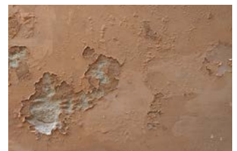
Damage to wall caused by flooding.
